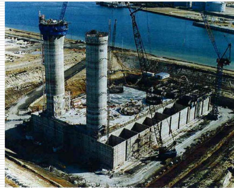
Construction of Shafts
