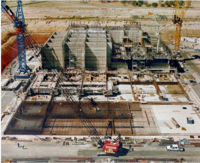
Construction of Base Slab
