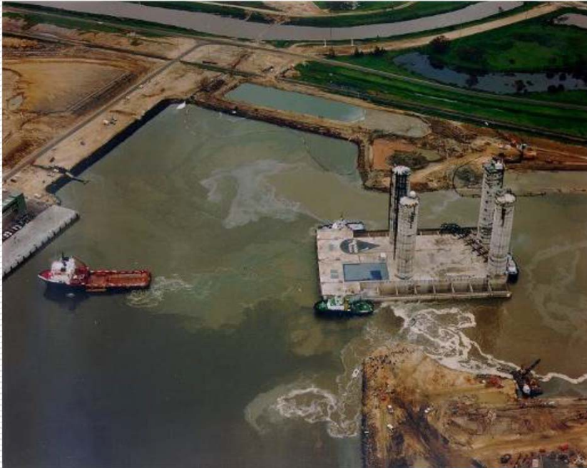
Float-out from casting basin
