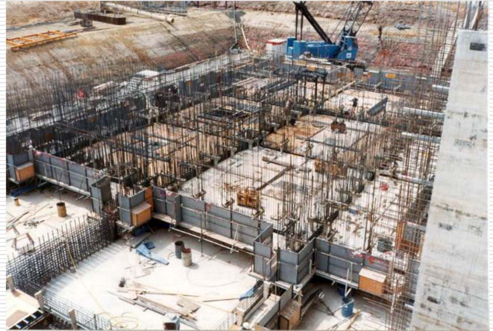
Construction of Base Caisson Walls
