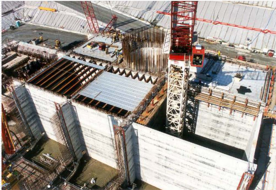
Construction of Roof Slab
